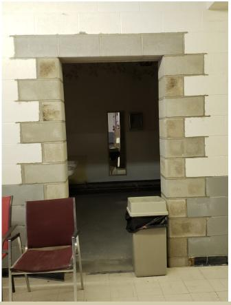
Work is coming along on the women's restroom in the basement. The old doorway has been closed up with wall bricks. A new doorway (above) has been made to accommodate a handicap-accessible stall which will be coming soon.
